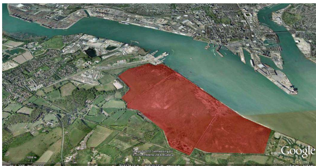
Figure 2-10: Aerial View of Southampton (Dibden Bay)
