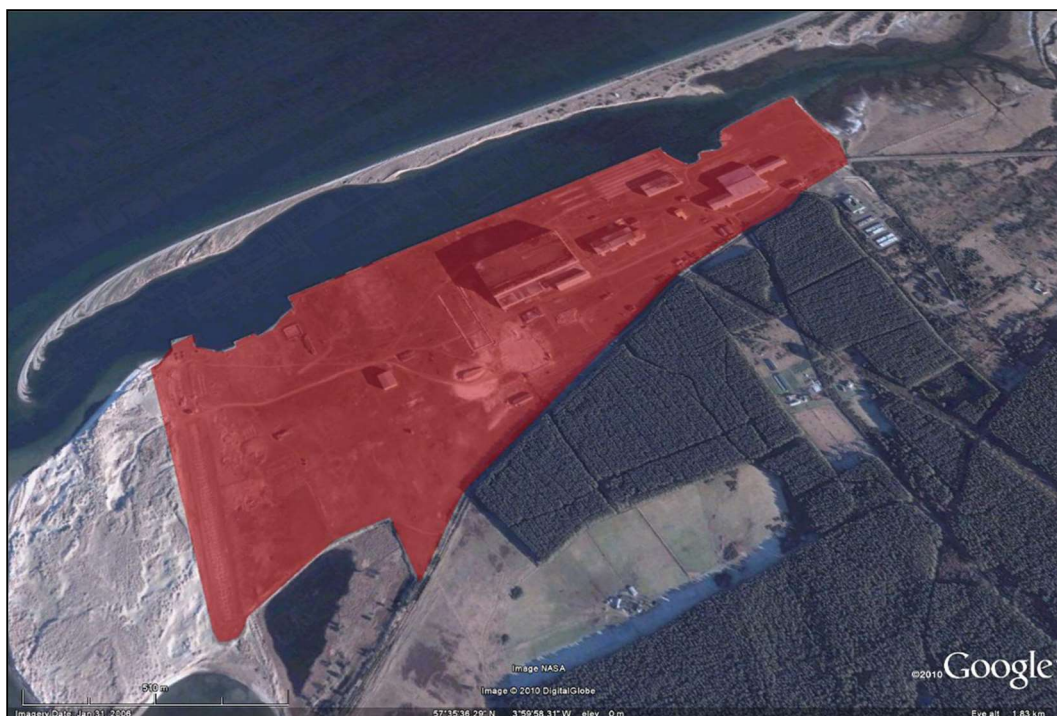
Figure 2-5: Aerial view of Ardersier
